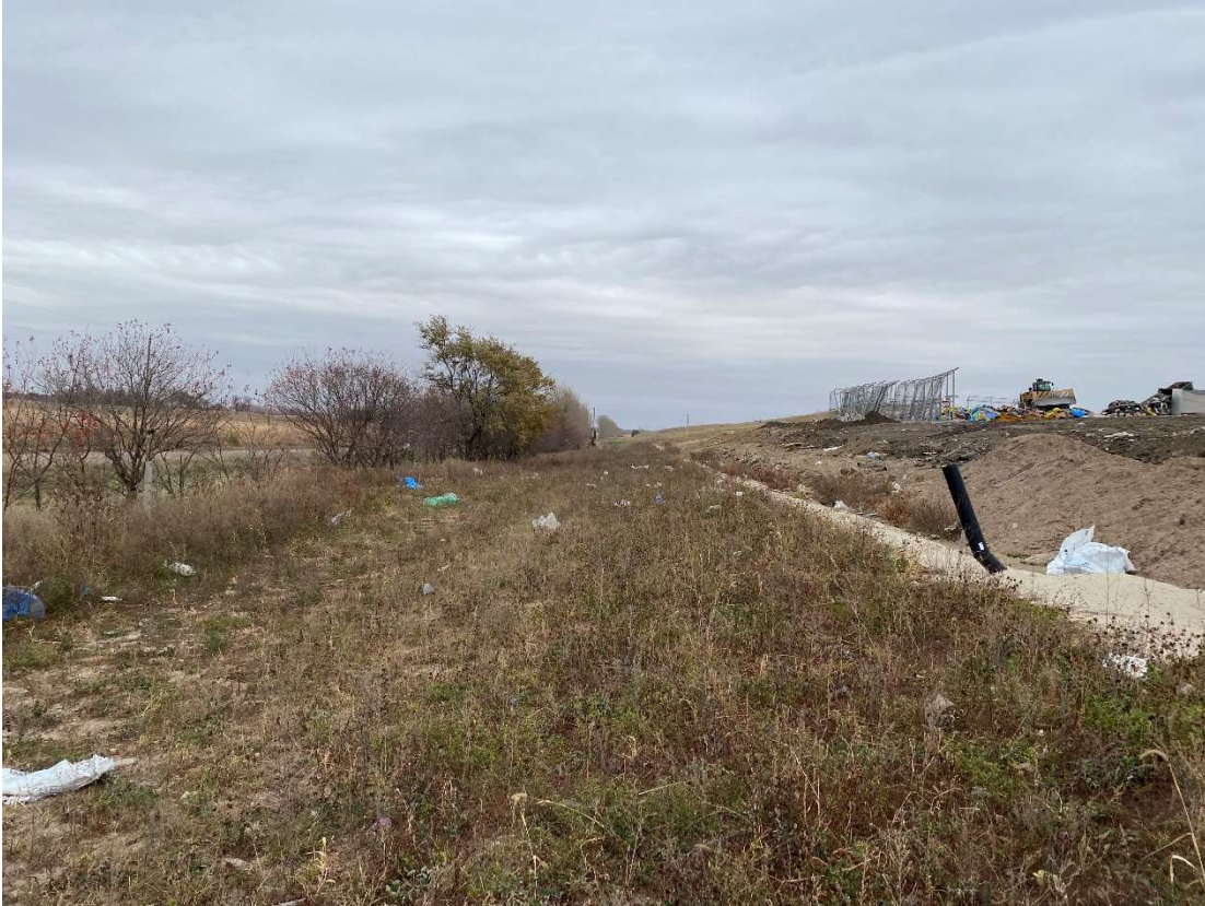
Location 14 – Looking East, Phase 5 Toe of Berm
