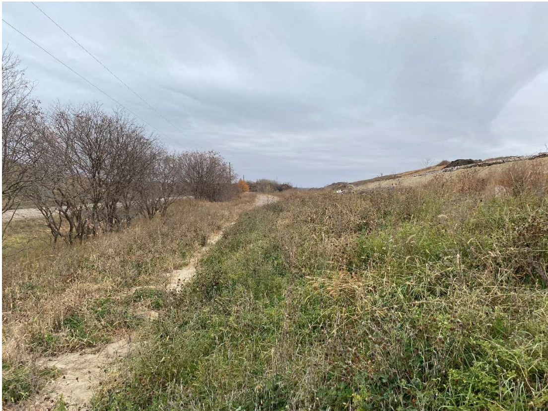
Location 13 – Looking South, Phase 5 Toe of Berm
