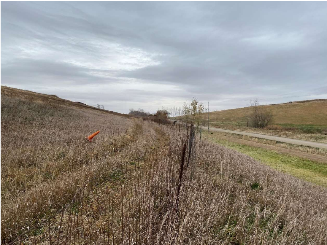
Location 8 – Looking North, Phase Eastern Berm
