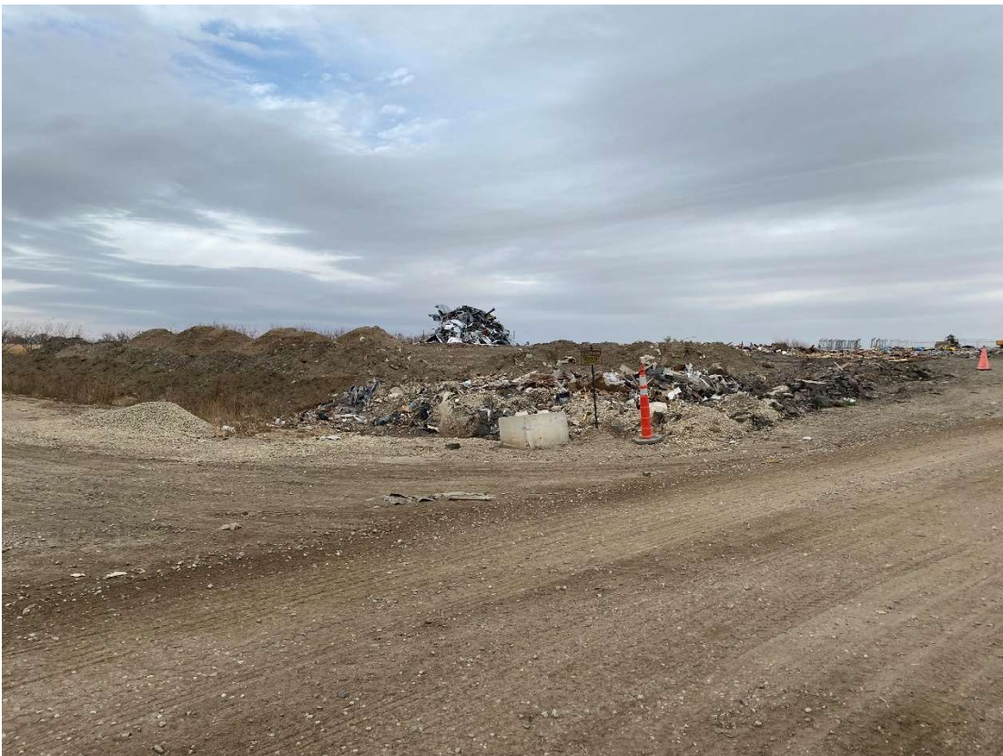
Location 2 – Looking Northeast, Phase 4 Anchor Trench
