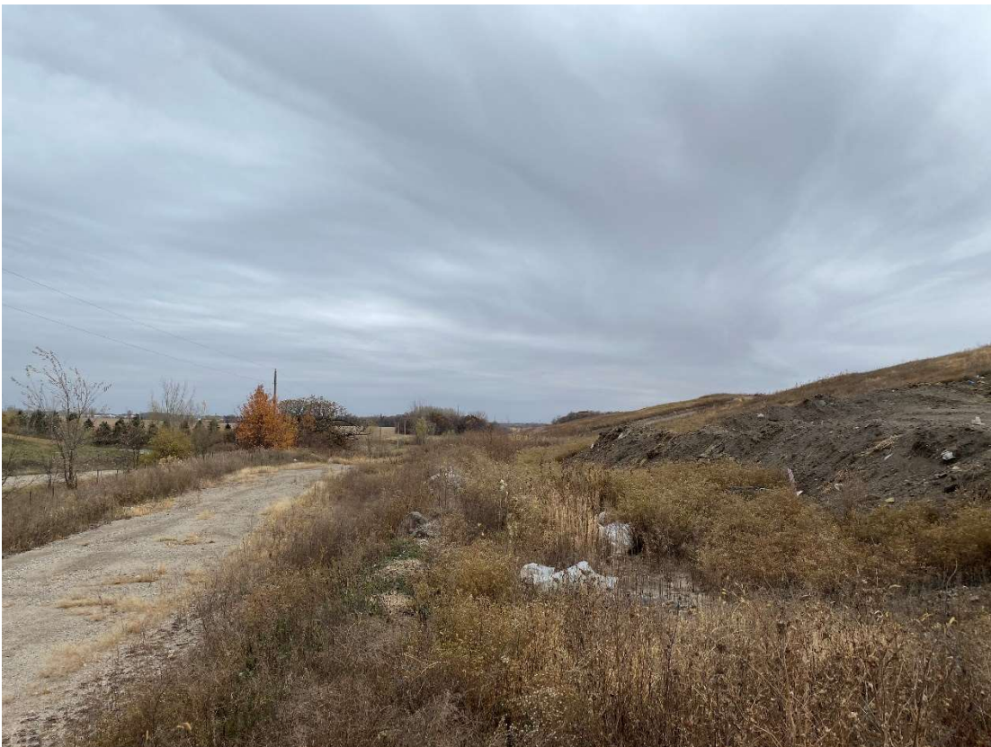
Location 11 – Looking South, Phase 4 Eastern Anchor Trench
