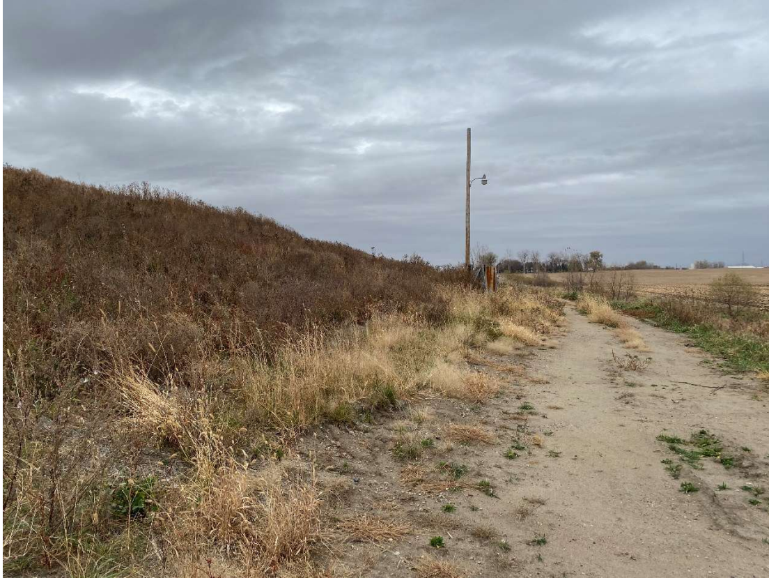
Location 6 – Looking East, Phase 2 Southern Slope
