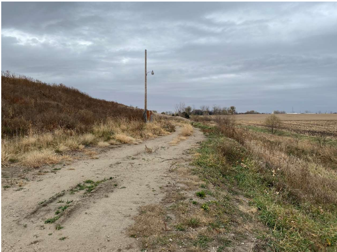
Photo 14: Location 6 – Looking East, Phase 2 Southern Berm
