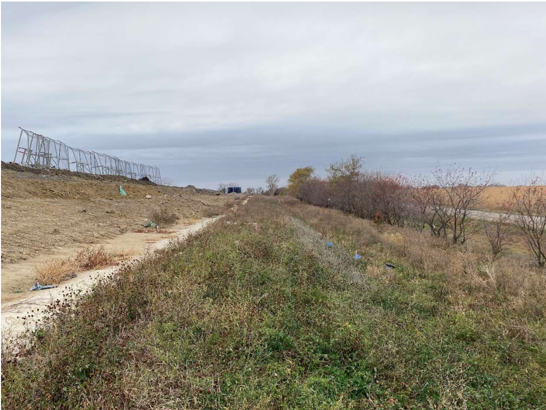
Location 13 – Looking West, Phase 5 Toe of Berm
