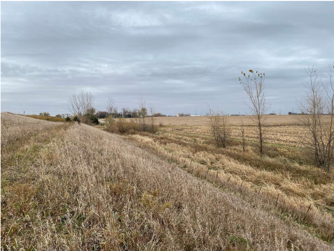
Location 7 – Looking East, Phase 2 Southern Berm
