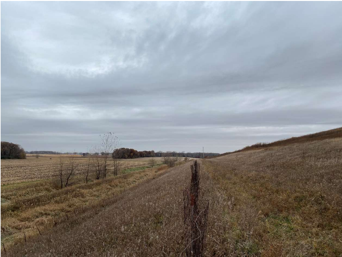
Location 8 – Looking West, Phase 2 Southern Berm
